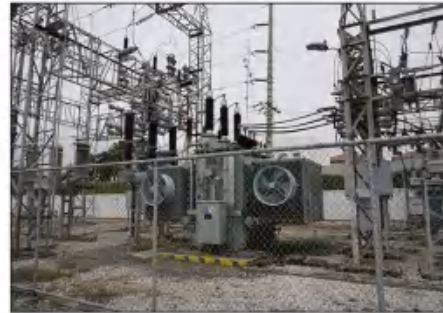
IEEE Standard 110KV Power Transformer in Solar Plant, Honduras
