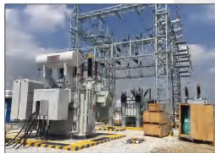
69KV Power Transformer in Power Substation, Ecuador
