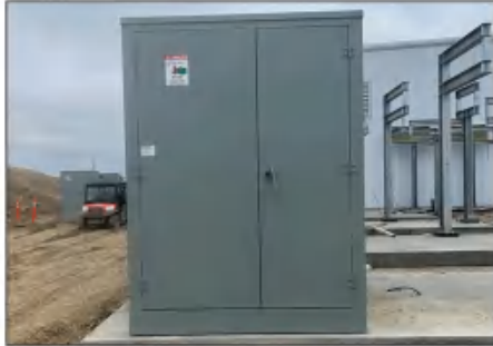
Three Phase Pad Mounted Transformer in Bitcoin Project ,Texas in USA
