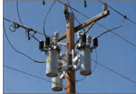
Single Phase Pole Mounted Transformer operating in Canada
